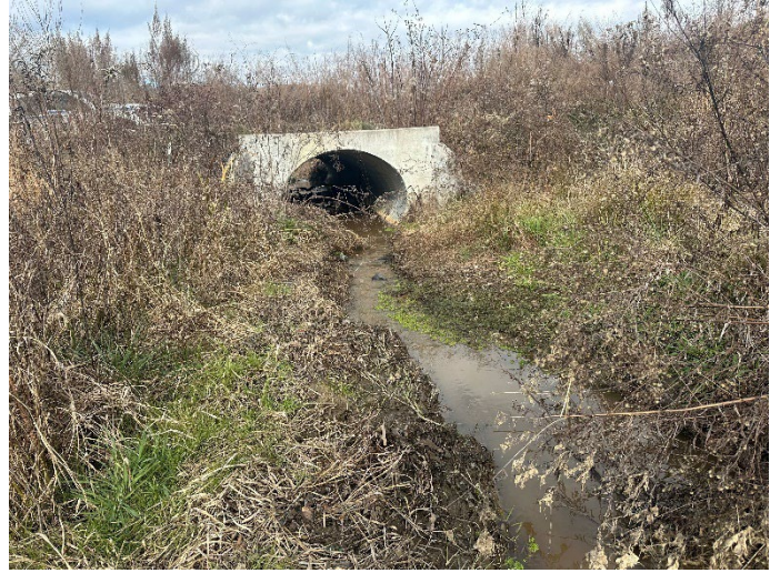
Supplemental Photo PP2 Area Downstream
